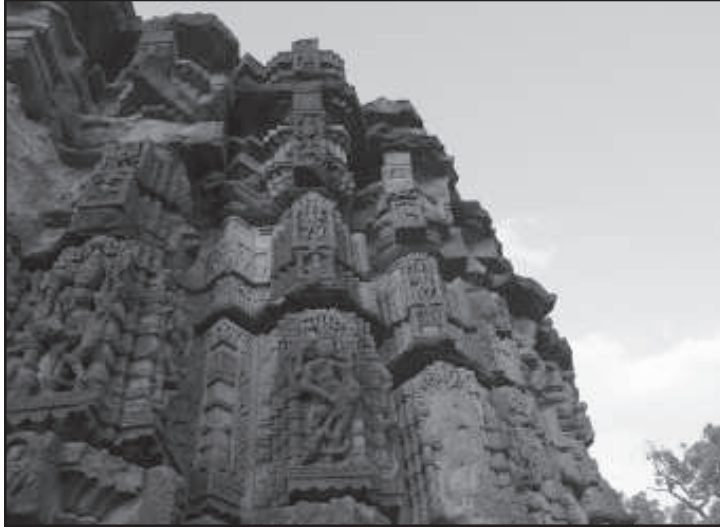
Fig. 6: Close view of the bhitti-shikhara , transition towards Bhumija (Courtesy: Snehal Joshi, Nashik)
